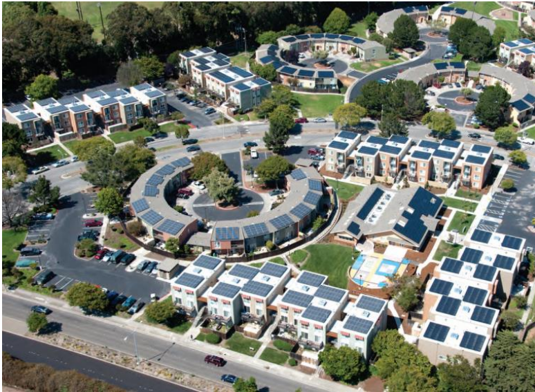
Figure 3. Multifamily installation at Crescent Park, Richmond
