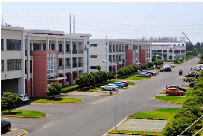
Wujin National Hi-Tech Industrial Zone, China
