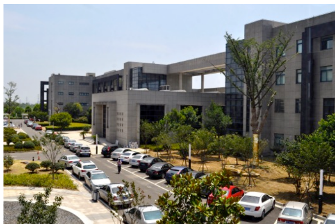
Wujin National Hi-Tech Industrial Zone, China
